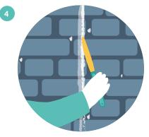
Shape the jointing compound to suit as it begins to go firm. The putty knife can also be used to apply the filler if required.
