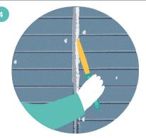
Shape the jointing compound to suit as it begins to go firm. The putty knife can also be used to apply the filler if required.
