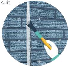
5 Introduce final texture to jointing compound with brush dipped in cleaner
