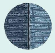
Corners - Raise /lower panels to align features. Mark position of corner, cut to form mitre. Fix panels leaving approx. 5mm gap, apply jointing compound and shape to suit
