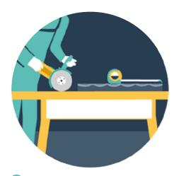
1 Measure, mark out and trim panels as required to align features
